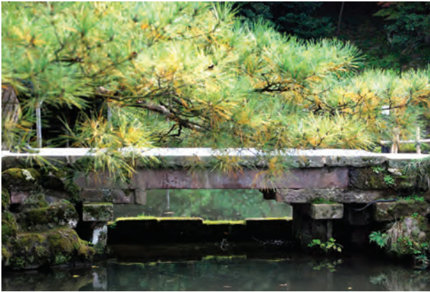
Concrete slab produces an interesting bridge.
